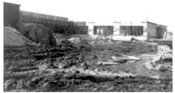
1st floor of the west wing during construction
