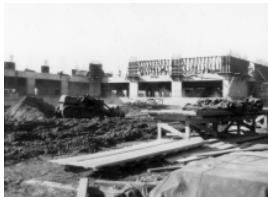
The 2nd floor of the west wing during construction
