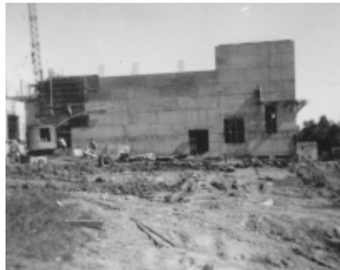
The south wall of the auditorium being built
